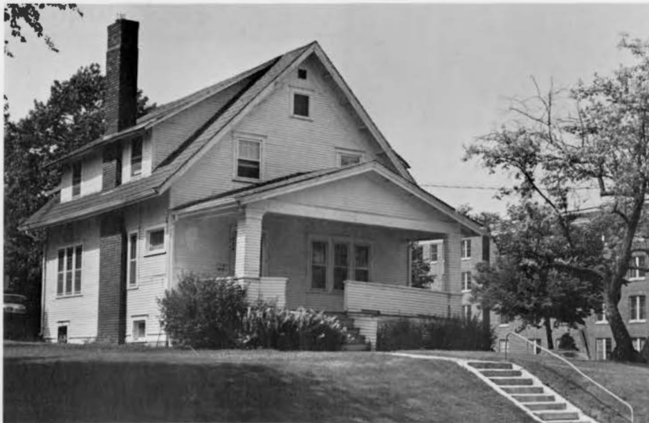
The Microcomputer Curriculum Project house, located across the street from Campbell Hall, received a new roof and other repairs in August.
