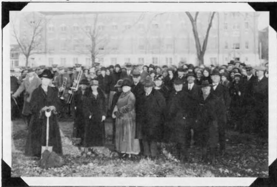
Breaking ground for the Campanile - 1924
