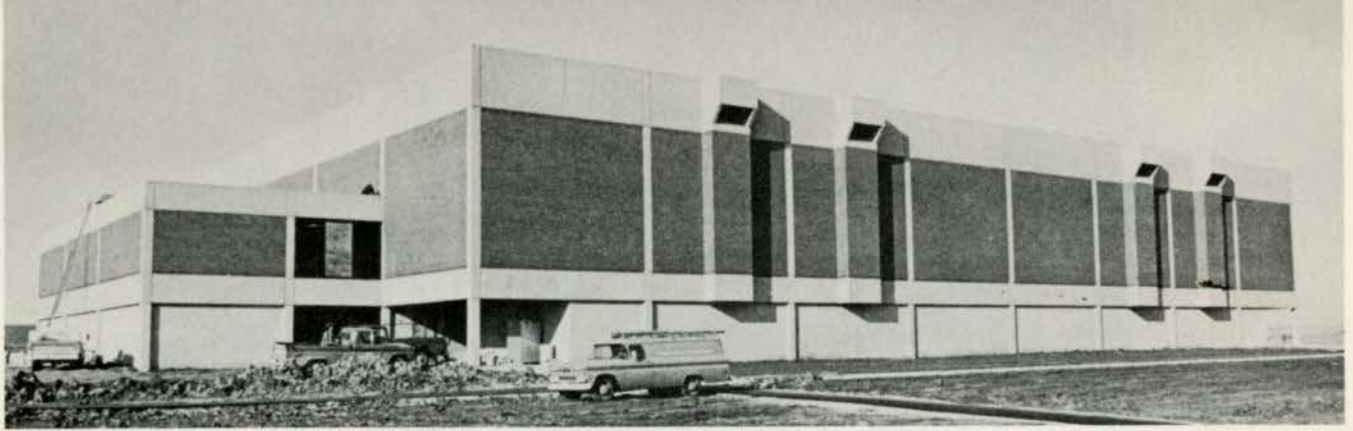
The new Physical Education Building, soon to be ready for use.
