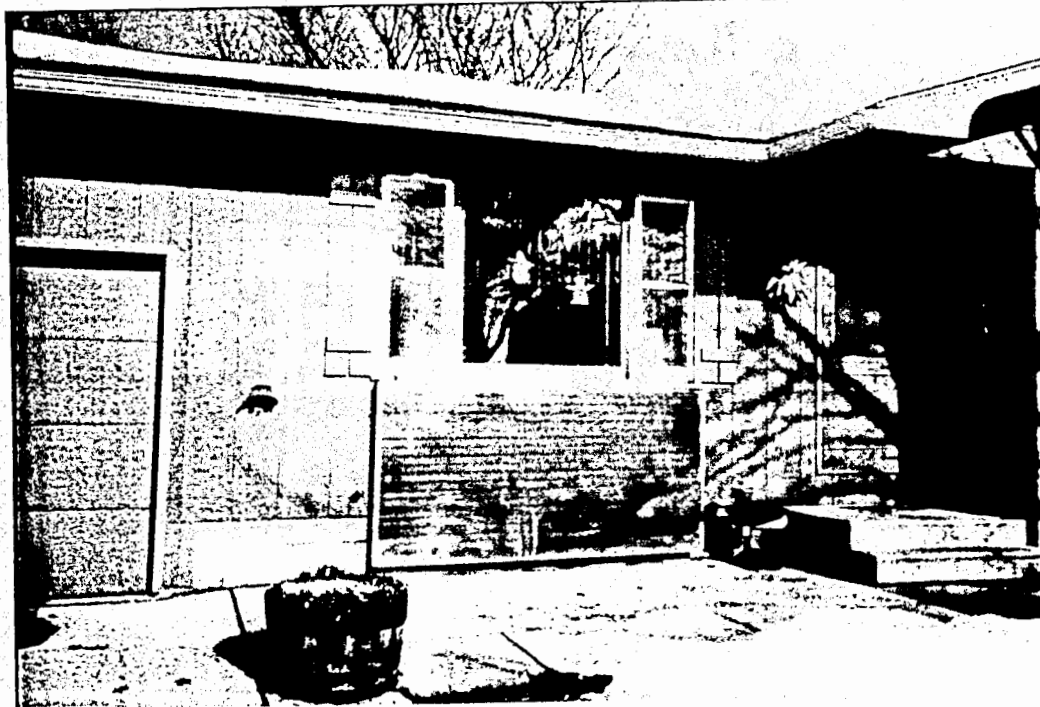
Flush-mounted SRRS at second test home Lovejoy
