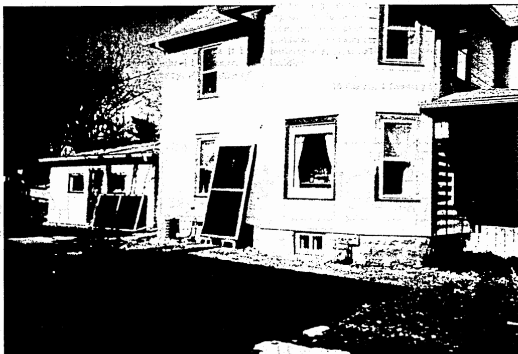
Vertically-angled SRRS at Washington; previously-used collector purchased at garage sale
