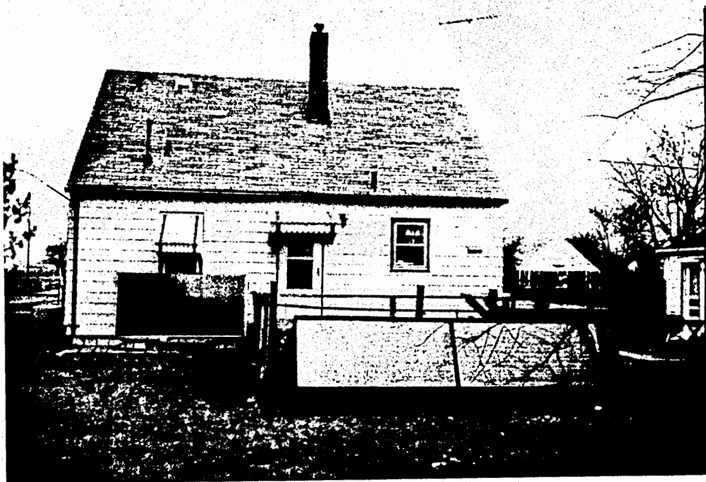
First installed SRRS and combination air/water collector constructed with recycled materials at test home North
