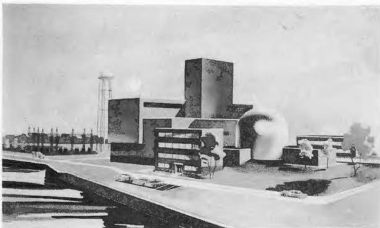
Figure 10 is an artist's concept of the final plant and shows the steel-domed reactor building. The building is 72 ft. in diameter, has an overall height of about 120 ft. It is set about half below ground. It is designed to contain all radioactivity in the event of an incident and can withstand an internal pressure of 32 psig at 650° F.
