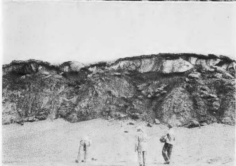
Figure 5. View of beach used as road at Barrow Base. Note "weasels" and deep ruts in low bearing capacity gravels. The deeper ruts are made by jeeps and trucks.
