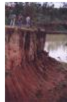
The edge of a previously mined area.
