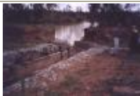
Heipang gullies were built by the government to stop erosion caused from abandoned tin mining sites.
