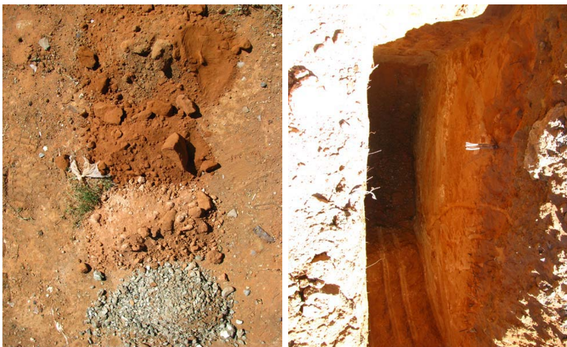
Figure F.7: Test pit 2 materials and test pit
