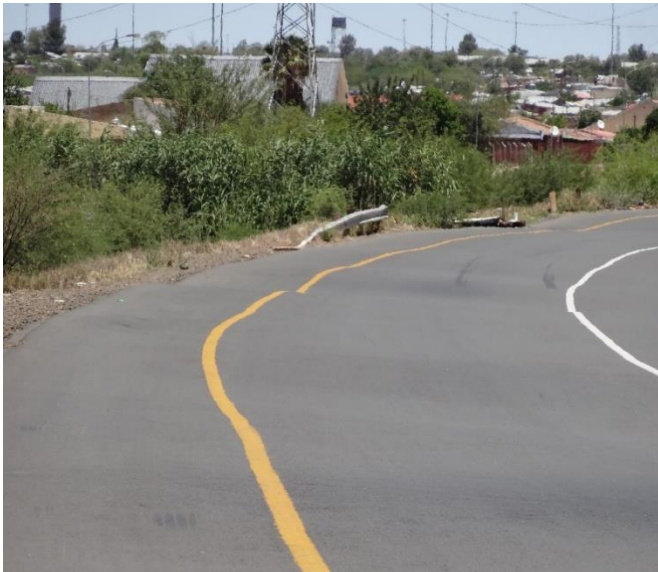
Figure 14 Undulations in a road close to a housing project where heave damage occurred and variability in suction potential was found to be substantial
