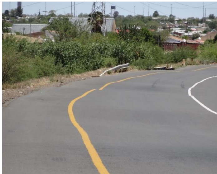
Figure 7.14: Undulations in road.
