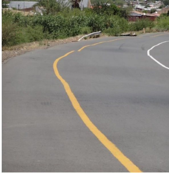
Figure 1.6: Undulations in a road.
