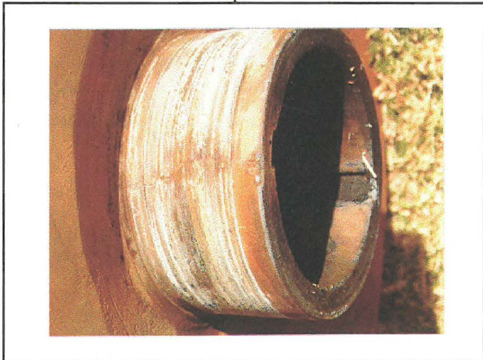
Figure 5-83: Picture shows cracks on the impeller shroud
