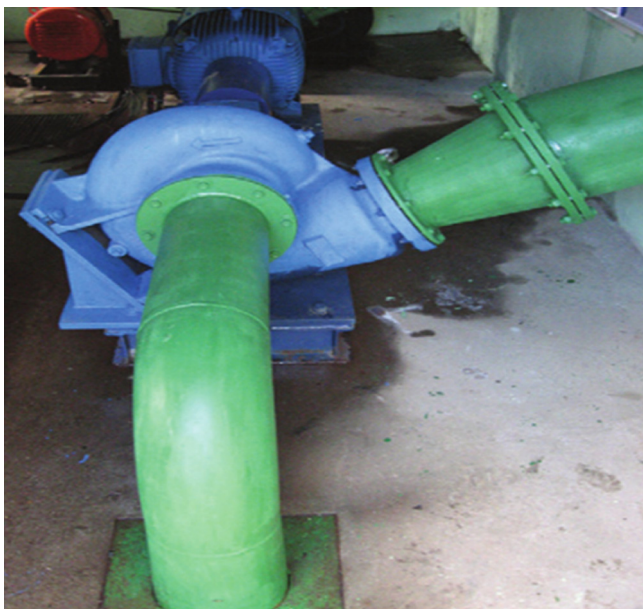
Fig. 2. Installed pump as turbine [23].
