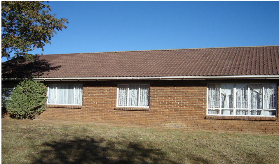
Figure 3.3 Case study House – Western facade.
