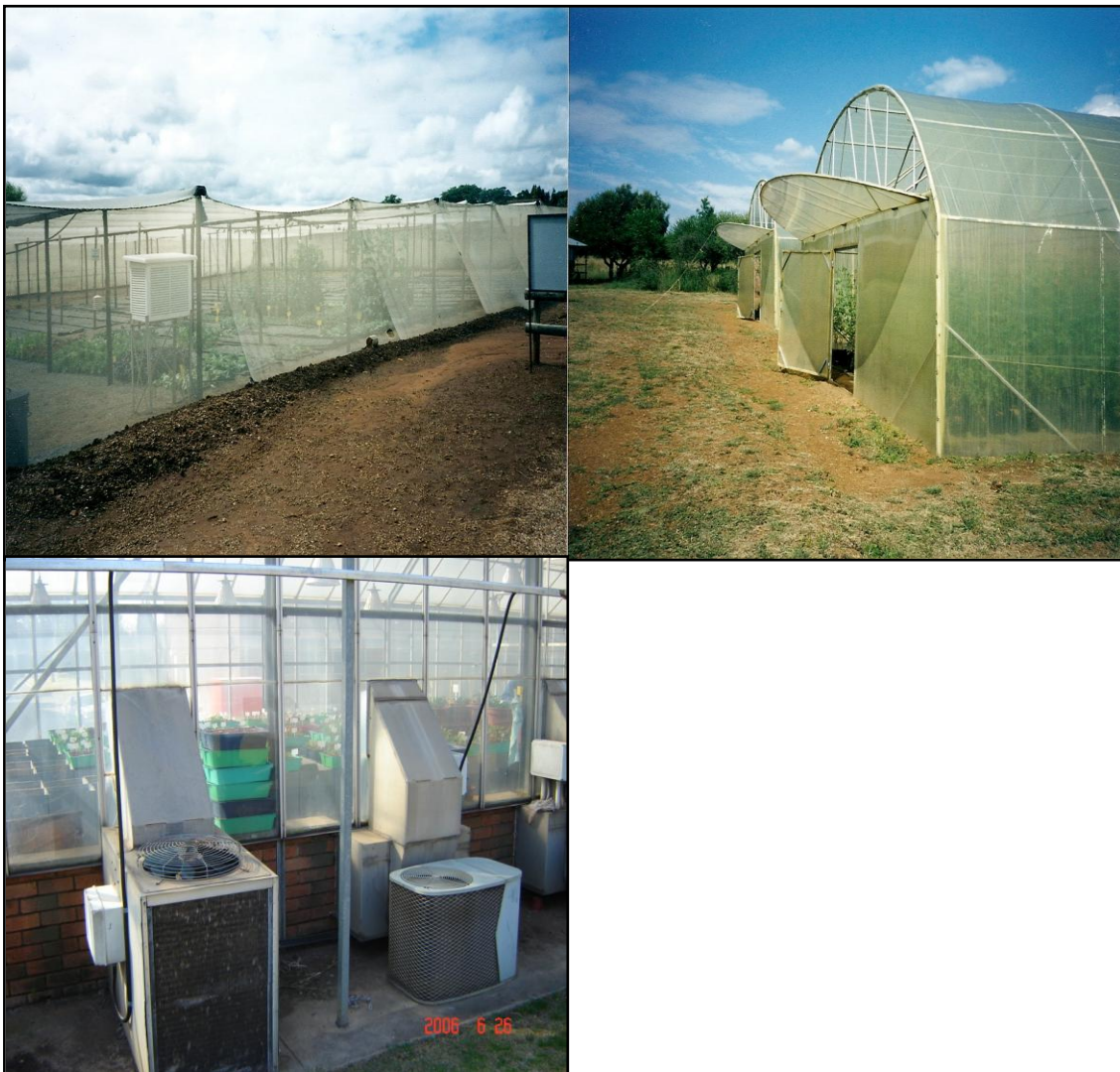
Figure 1.2: Most important protective structures used in the production of certain crops. Shadehouse structure (top left), plastic tunnel (top right) and glasshouse (bottom).
