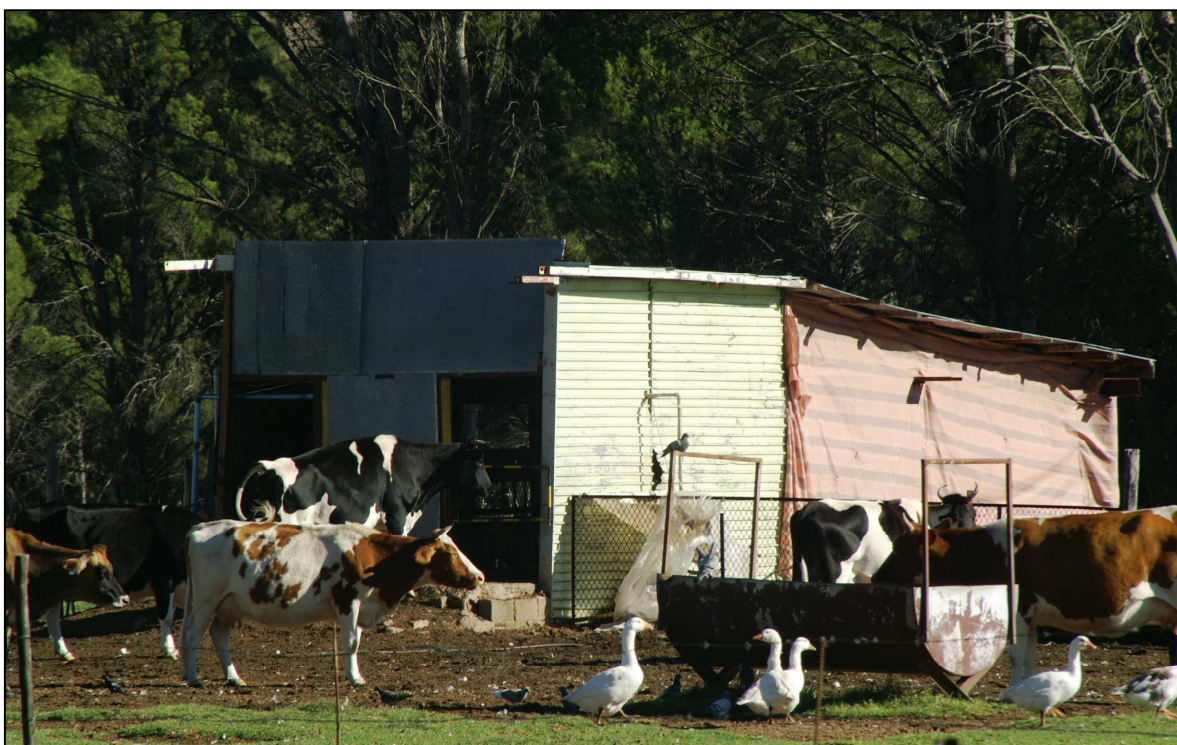
Figure 4.3: Unregistered milking shed in a structure that does not comply with the minimum statutory requirements in accordance with regulation 1256 of 27 June 1986, where milk is produced for human consumption as described above and sold at their roadside stall as depicted in Figure 4.4.
