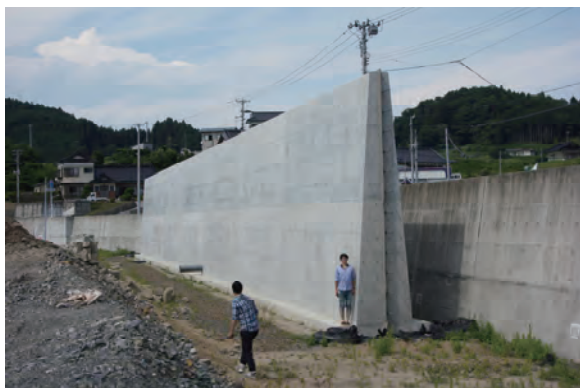
Figure 5 The seawall in Rikuzentakata, Iwate Prefecture
