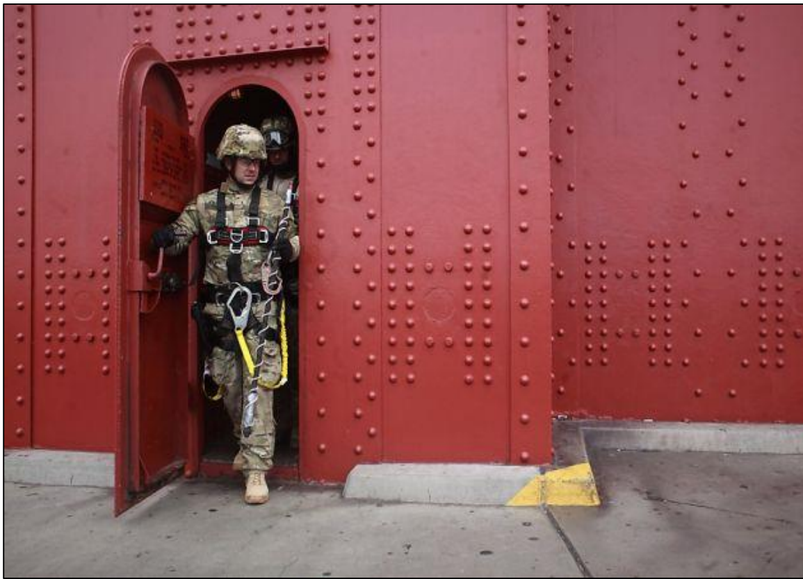
Fig. 1-6: Riveted Golden Gate Bridge South Tower (photo from SFGate, at http://www.sfgate.com )
