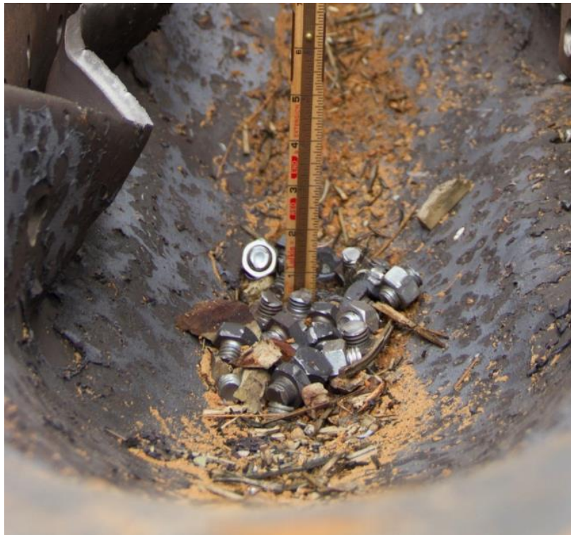
Fig. 3-2: View of Bolts Shear Failure Following Testing (from Crane et al., 2015)
