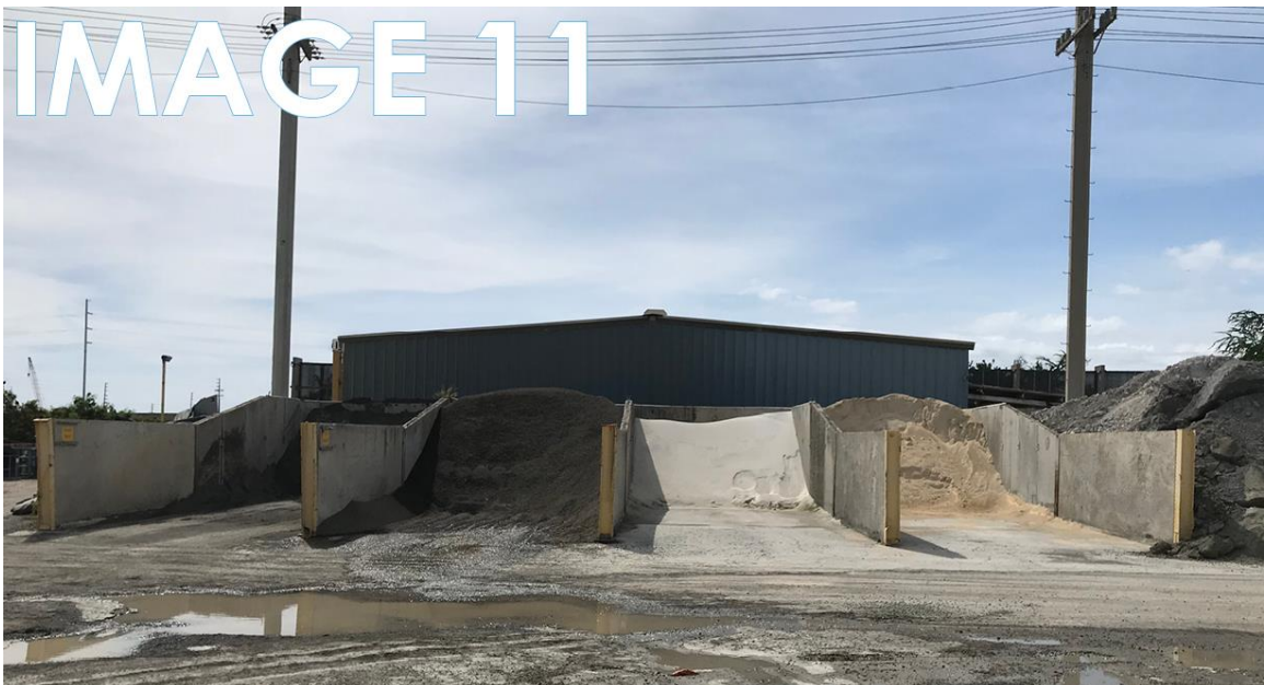
Figure 39: Aggregate Piles 2 Source: Author
