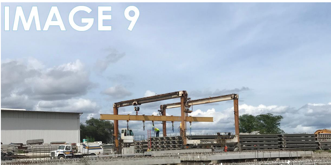
Figure 37: Large Crane and Pulley System Source: Author
