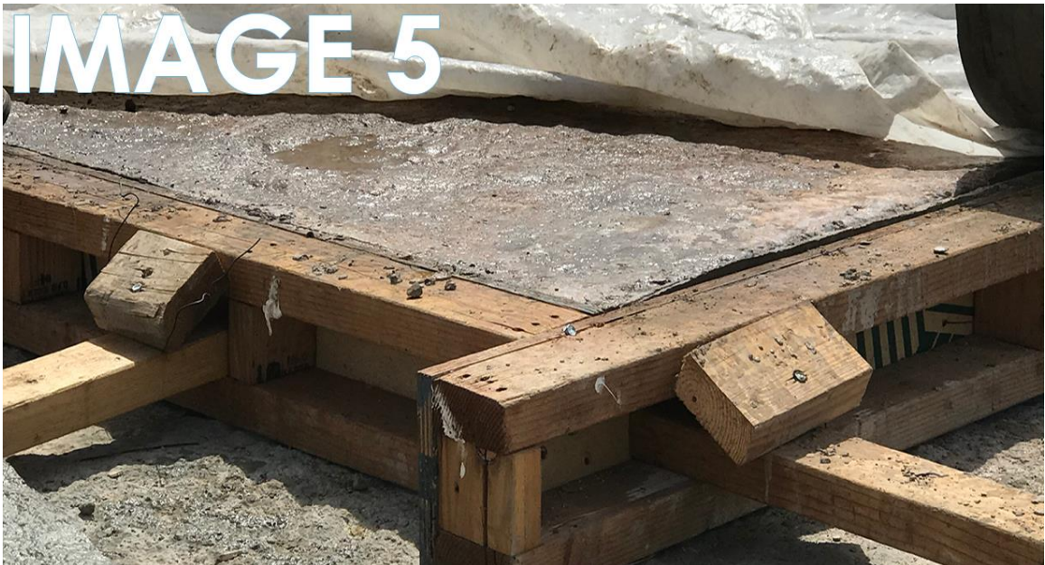
Figure 33: Precast Concrete in Wood Form Source: Author
