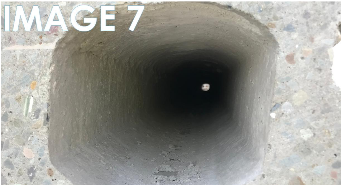
Figure 35: Precast 8" Hollow Core Units 2 Source: Author
