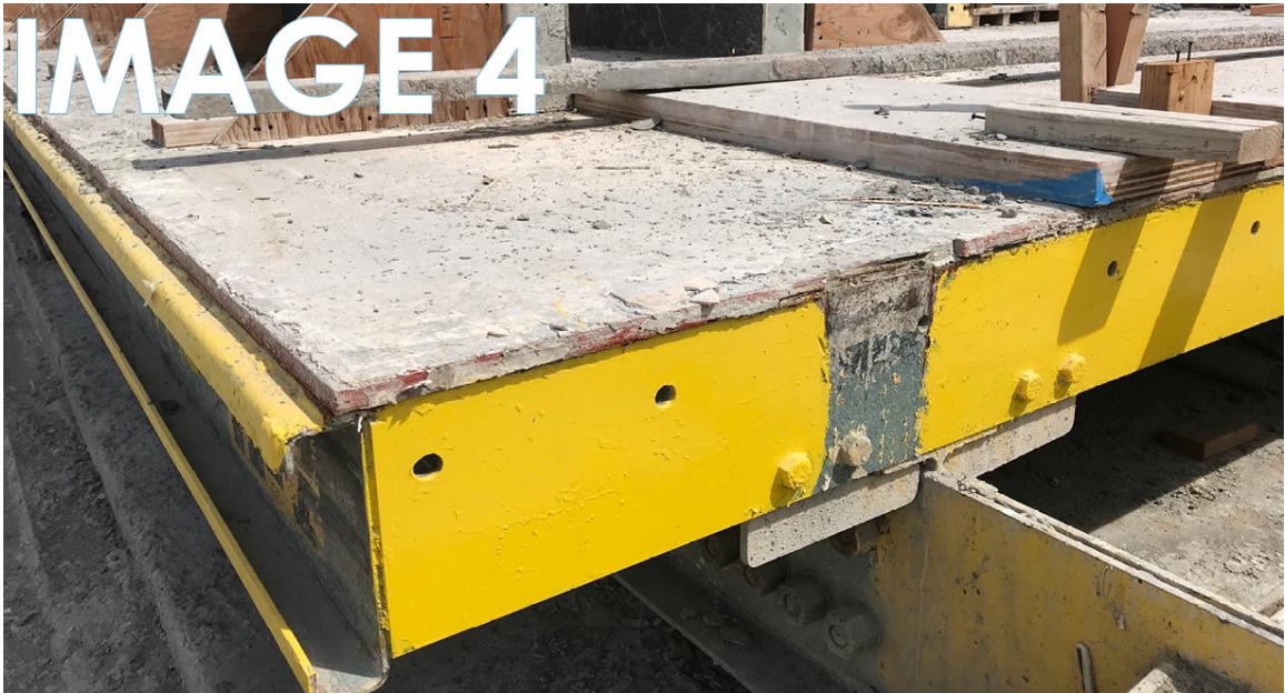
Figure 32: Precast Concrete in Steel Form Source: Author
