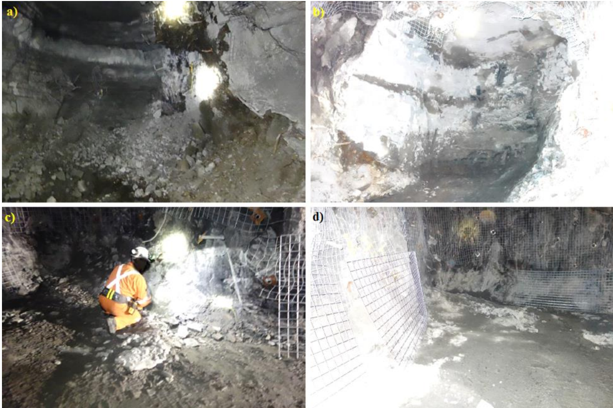
Figure D-2 Mine A misfires and underbreak: a) heading not cleared out, underbreak b) four missed holes c) three missed holes, d) 2.5ft floor heave that needs to be blasted before bolting
