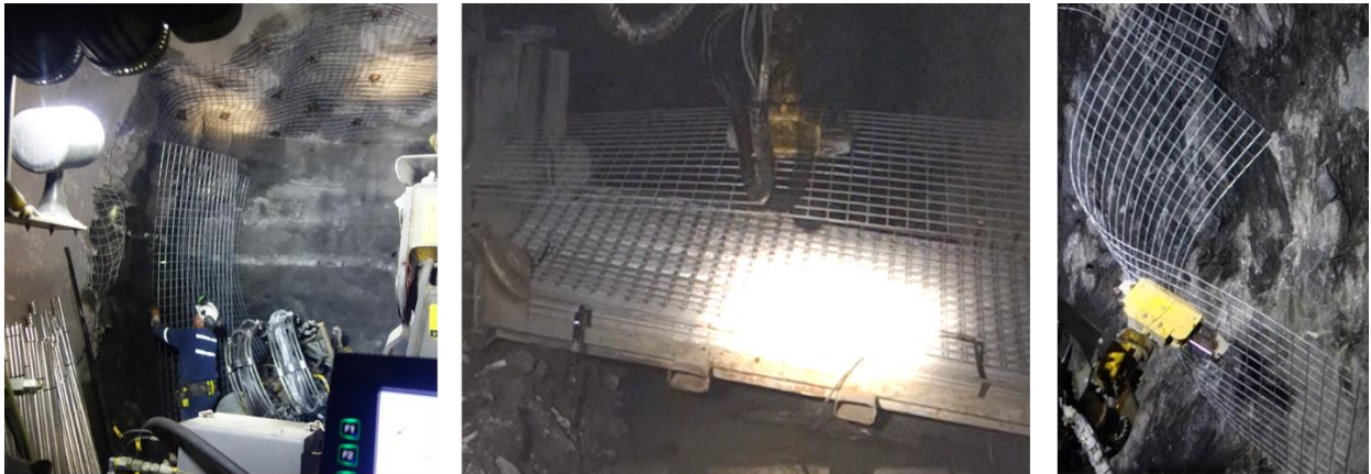
Left: operator installs screen manually, Middle: screen handling from bin Right: screen is dropped from the screen handling arm
