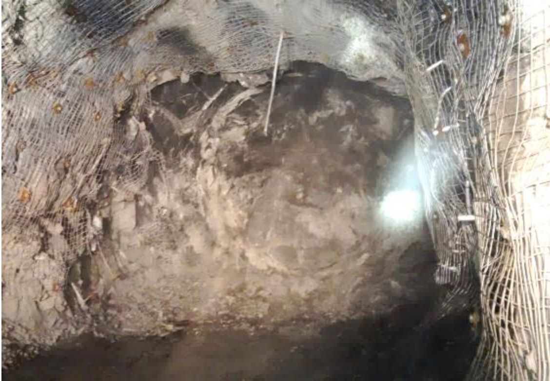
22ft x 22ft, 8ft deep unbolted heading
