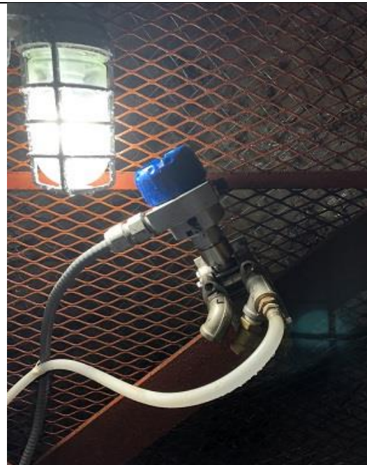
DPT2 – Differential pressure sensor
