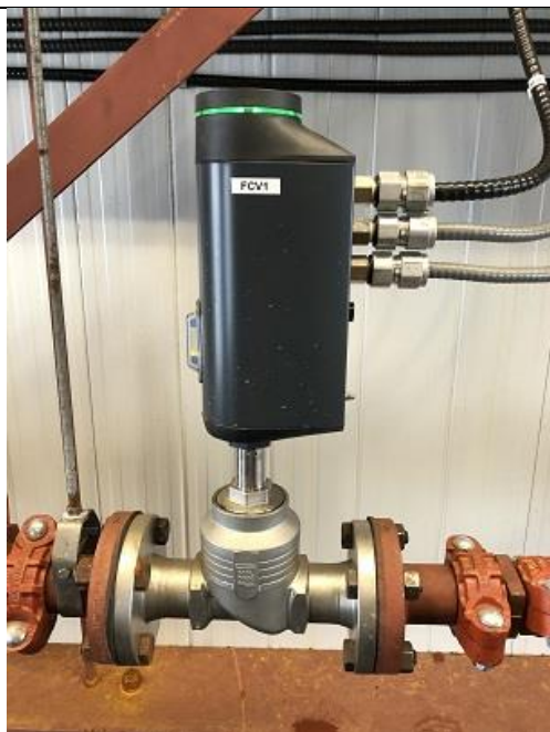
MCV – Motorized control valve
