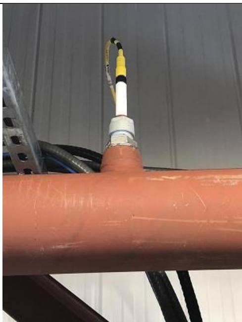
TT1/GT1 – Temperature and humidity sensor
