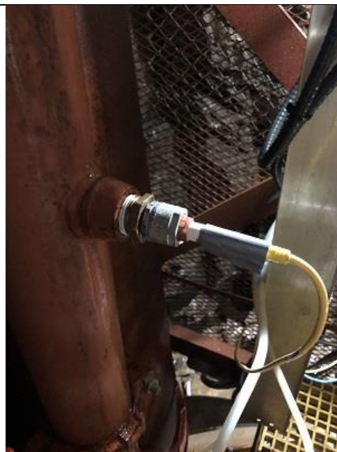
TT2/GT2 – Temperature and humidity sensor
