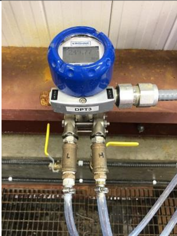
DPT3 – Differential pressure sensor
