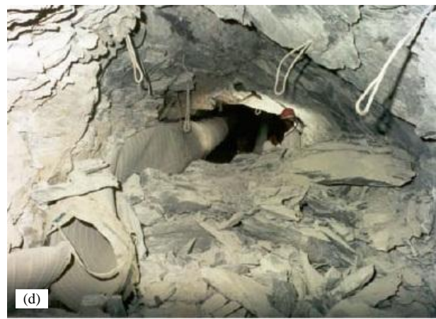
Figure 1-1: Examples of rockburst damage in deep tunnels at: (a & b) Brunswick Mines, Canada (White and Rose, 2012), (c) Jinping II hydropower station, China (Jiang et al., 2010), and (d) a mine in South Africa (Stacey and Rojas, 2013).
