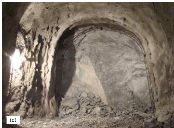
Figure 1-1: Examples of rockburst damage in deep tunnels at: (a & b) Brunswick Mines, Canada (White and Rose, 2012), (c) Jinping II hydropower station, China (Jiang et al., 2010), and (d) a mine in South Africa (Stacey and Rojas, 2013).
