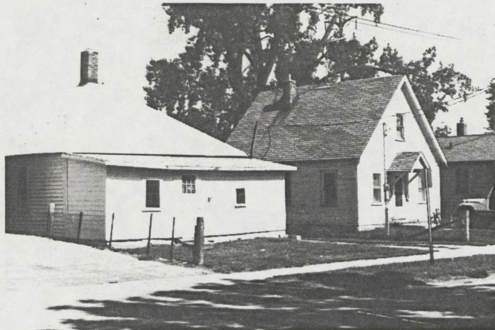
Examples of Rochester homes that meet substandard criteria.
