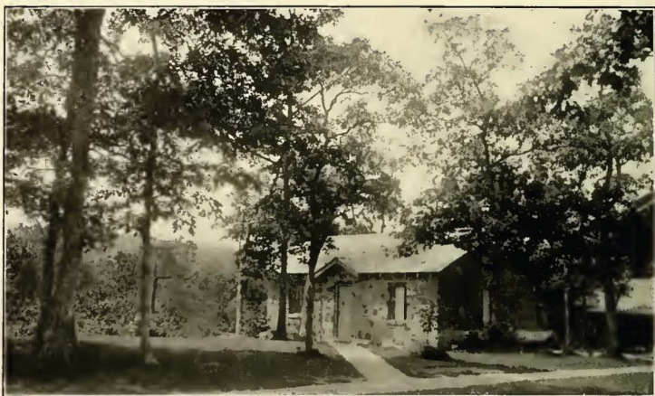
THE LIBRARY BUILDING, MOUNTAIN LAKE BIOLOGICAL STATION, MOUNTAIN LAKE, VIRGINIA.
