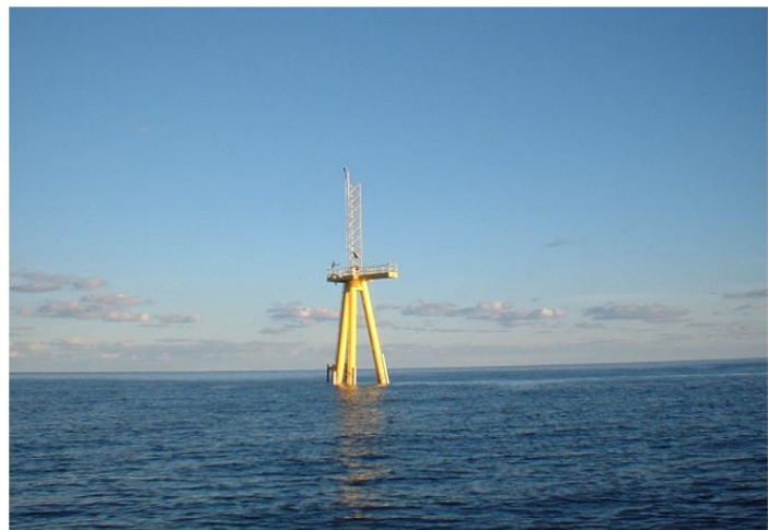
Figure 11: MVCO's existing Air-Sea Interaction Tower (ASIT) located 1.5 Nm offshore of the island of Martha's Vineyard. Facing predominantly onshore winds and open ocean wave - large fetch - conditions during the summer months, the ASIT was built to allow boundary layer studies. Image credit: WHOI.
