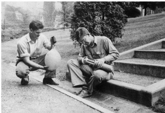
Figure 7. Worzel and Ewing assembling charge for submarine SOS location signal. (Courtesy of WHOI Archives)
