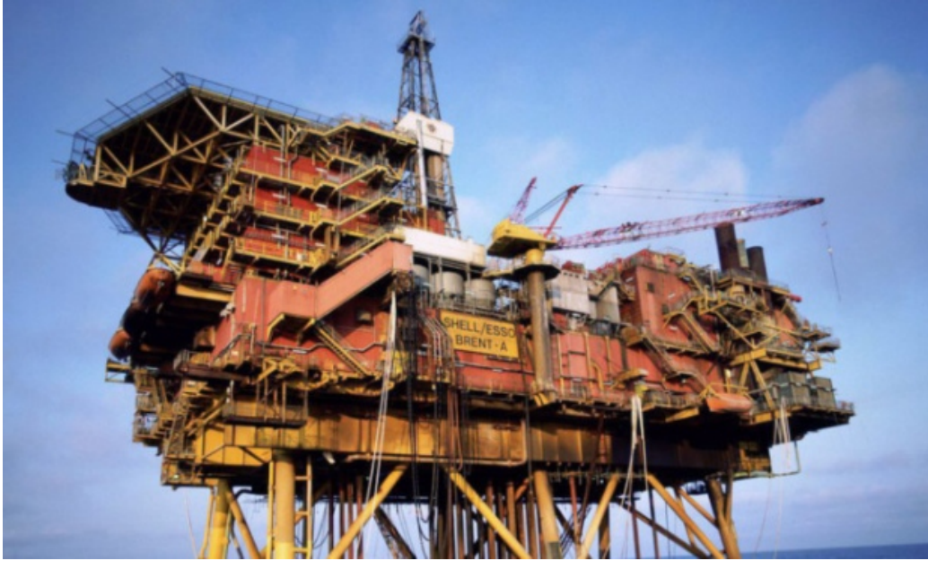
Figure 1-1: Topsides of a typical offshore structure in need of decommissioning [28].
