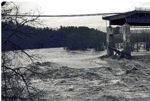
(a) Schoharie Creek bridge collapse, Fort Hunter, NY, 1987 (USGS)
