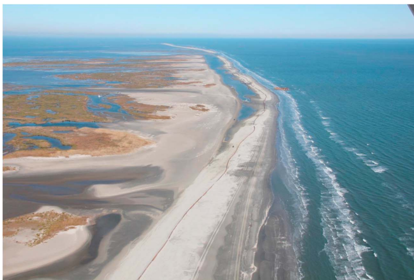
Figure 2. Construction of the Chandeleur Islands' berm (USGS Photo taken 22 January 2011).
