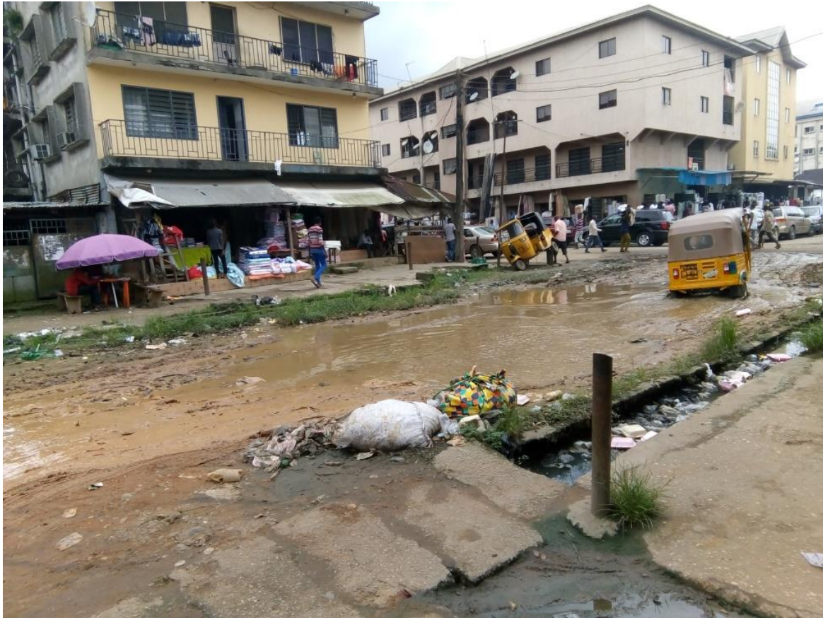
Picture 4: Indiscriminate dumping of refuse and dilapidated road in Aba [Credit: Researcher]
