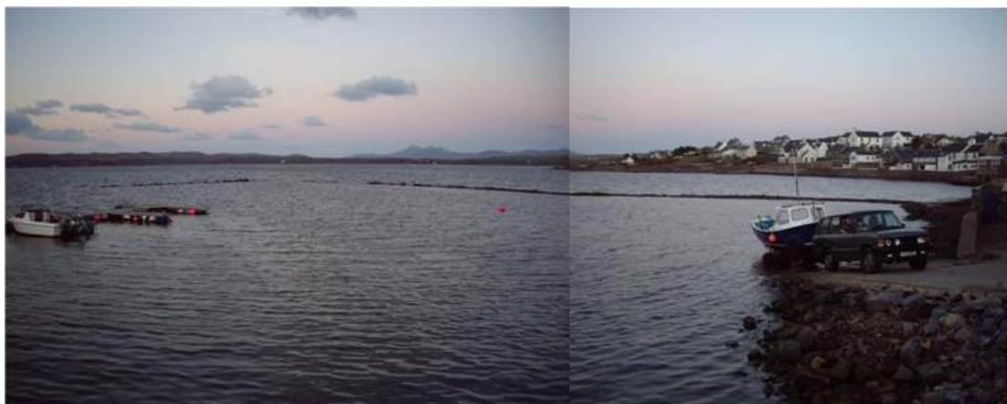
Figure 120 View of break water at high tide.
