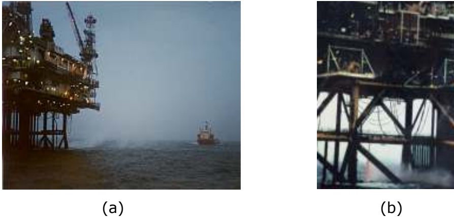
Figure 1 (a) Produced water discharge; (b) Tracer doped discharge
