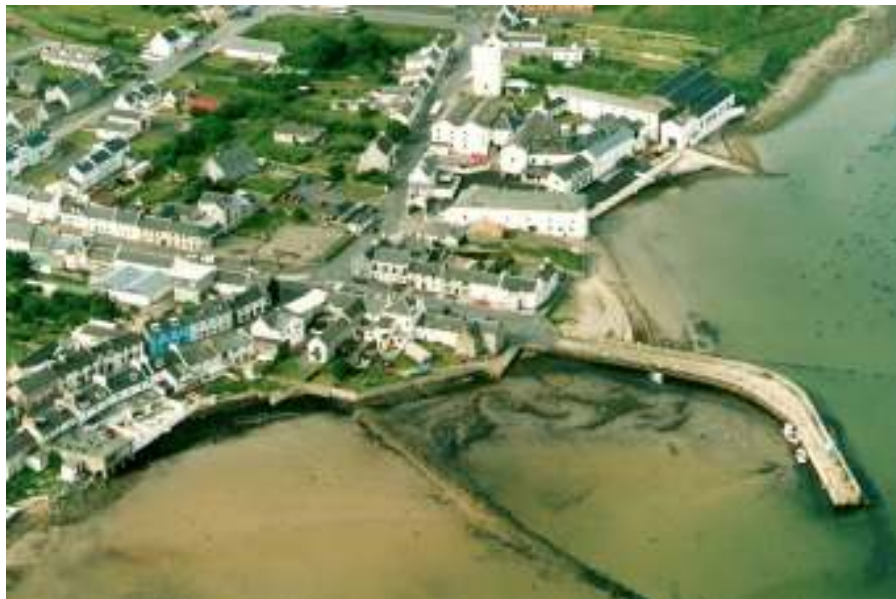
Figure 104 Bowmore Harbour showing silting
