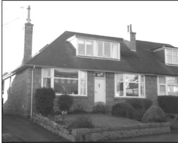
Figure 1: View of the house 1
