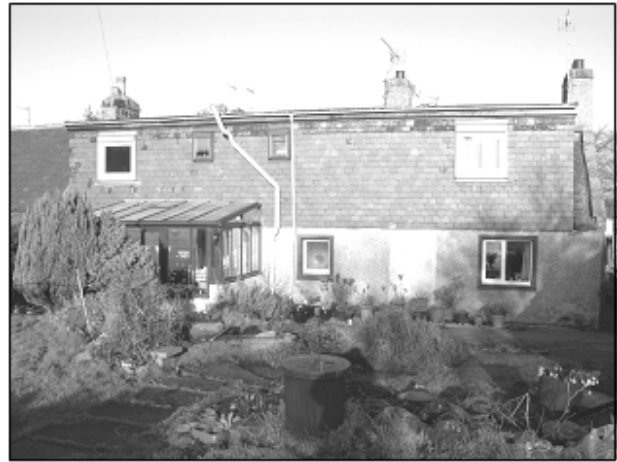
Figure 7: View of the house 2
