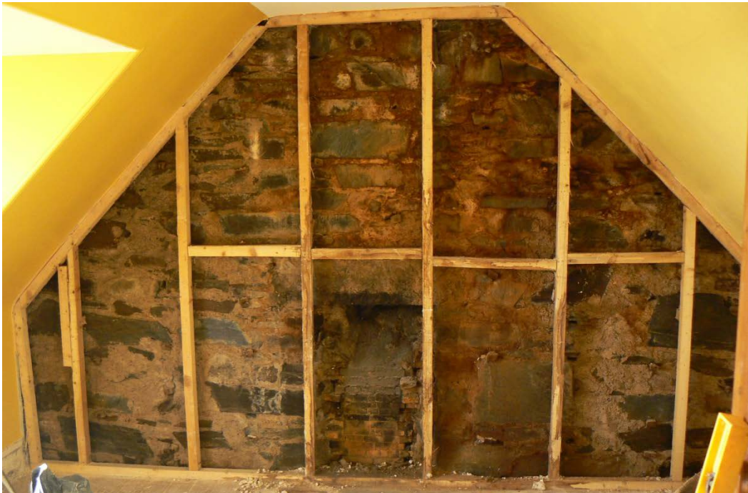
Figure 5. Use of insulation board internally.
