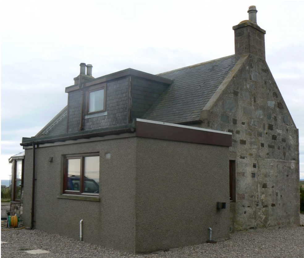
Figure 4. Solid external wall with internal lath and plaster removed.
