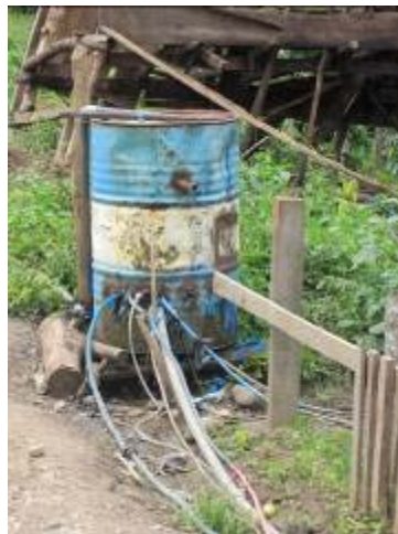
Figure 4-8: Terangengon water distribution system
