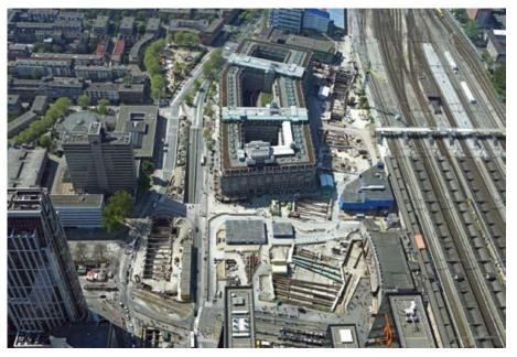
Figure 42 Work in progress. Left: the building pit for the new Weenatunnel. Right in front: the building pit for the underground
