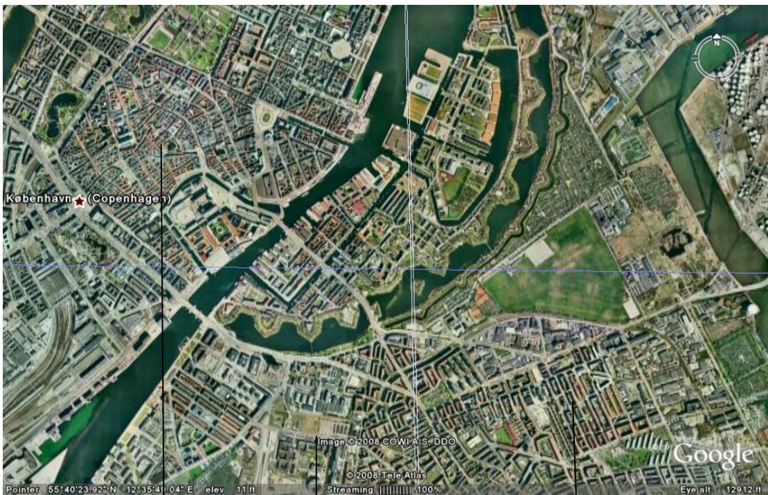
1. Old narrow town centre. 2. The new open area. 3. The one block building area.
