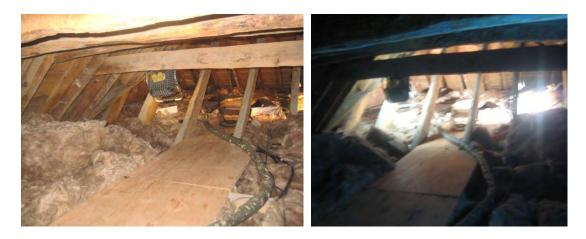
Floor covering and lighting installed for safety and easy access to the loft
