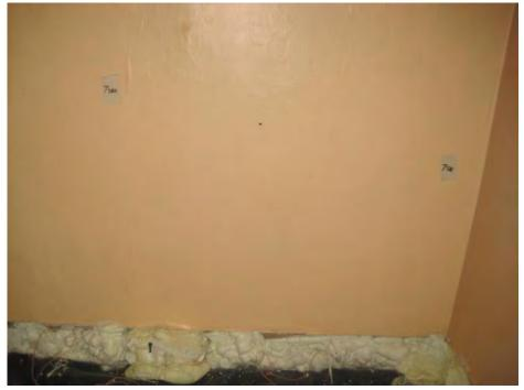
Leak of the foam at the bottom pat of the wall
