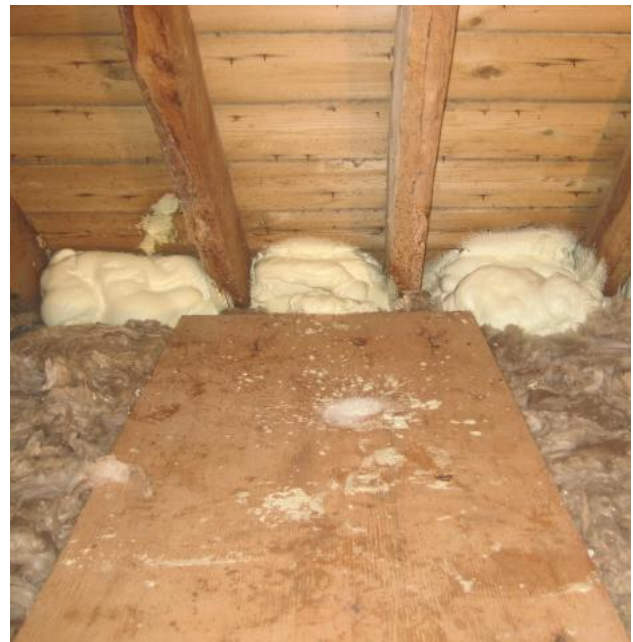
Figure 18. Foam seen at the eave level
