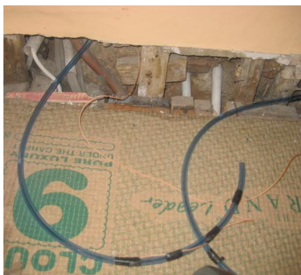
Figure 9. Pipes attached to cords
