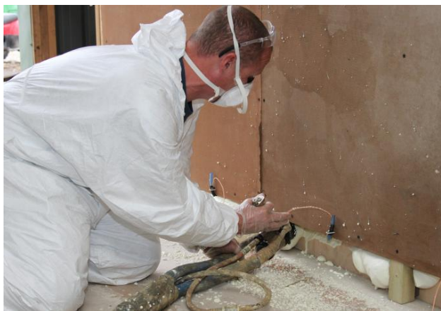
Figure 6. Injection of the foam
