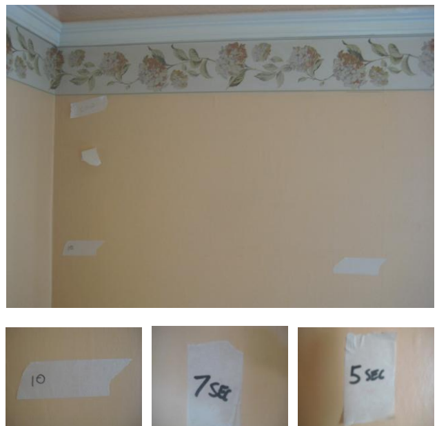
Figure 15. Alteration of bays and localisation of the foam level on the wall
