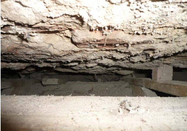
Figure 3. View inside the cavity wall before insulation
