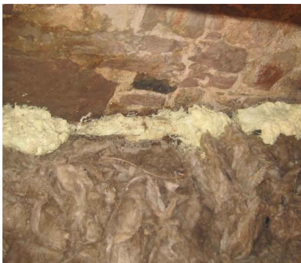
Figure 17. Top of the gable wall, foam seen from the attic
