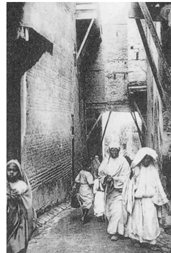
Figure 1.b: The cantilevered volumes constitute the means of a partially covered residential street (Source [1]).
