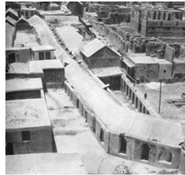
Figure 2.c: A semi-heavily urban roofing with openings located on parapet walls (Source [3]).
