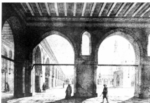
Figure 4: Various openings (open-spandrel arch naves and pierced tympanums) are used to maximise the penetration of daylight into the prayer hall (Source [7]).
