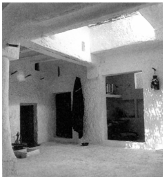
Figure 14: To catch the earlier sunrays, the women morning living room ( Izefri ), in the M'zab dwelling in Algeria, is often oriented to the south or southeast and is widely opened to the courtyard (Source: [20]).
