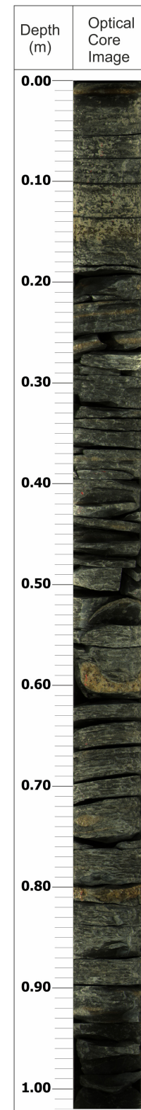
FIGURE 4 | Optical line scan image of a 1.02 m section of core from the Melbourne 1 borehole (985.66 m – 986.68 m) showing a large number of low angle fractures along bedding planes. Due to the condition of the core there was not sufficient coherent material to undertake UCS tests.
