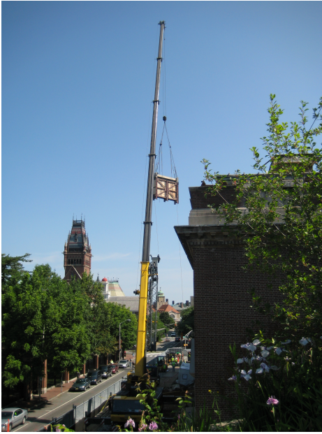
Figure 13 Crane removing Hunger March from the Fogg building, 24 June 2010. Photo: ©President and Fellows of Harvard College, photographed by the Straus Center for Conservation.
