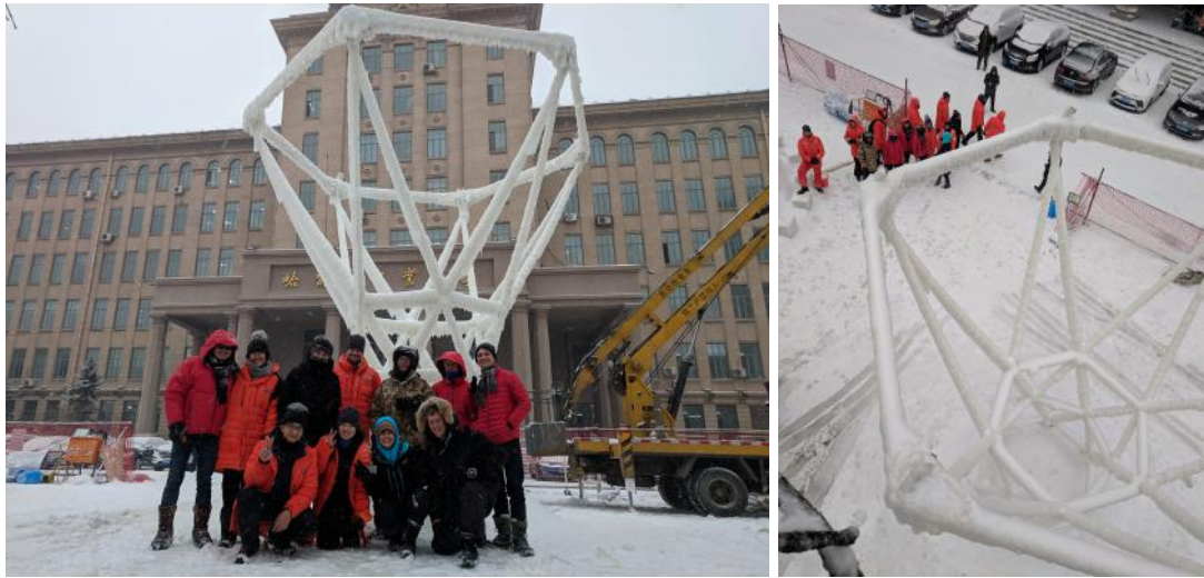
Figure 1: The team with the finished structure
