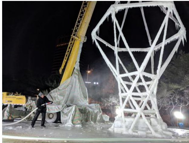
Figure 4: Spraying of the structure throughout the night
