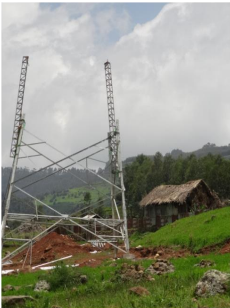
Electrical transmission line construction, Suluta area
