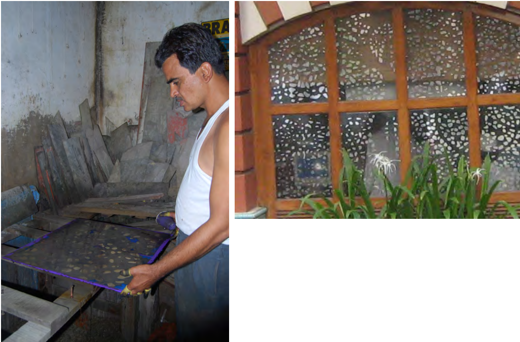
Images 9,10: Making window sections with Gamlish, and final installation at House of MG, Ahmedabad, 2007
