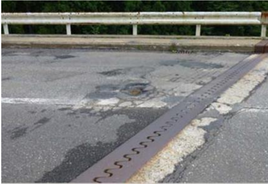
(b) The state near the joint of bridge
