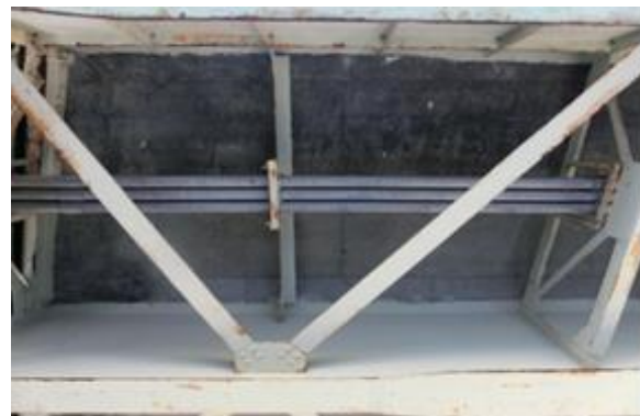
Figure 3.19: Deterioration of bridge deck
