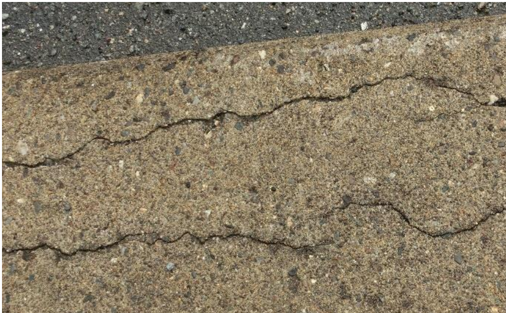
(a) Concrete wheel guard
