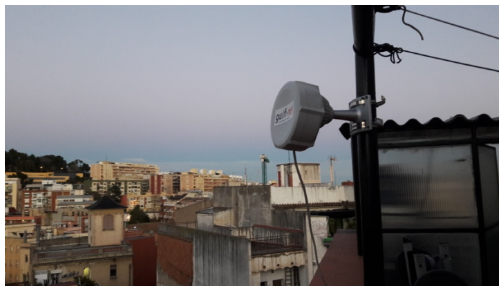
Figure 2: An individual “node” or connection point receiving a signal from a supernode.
