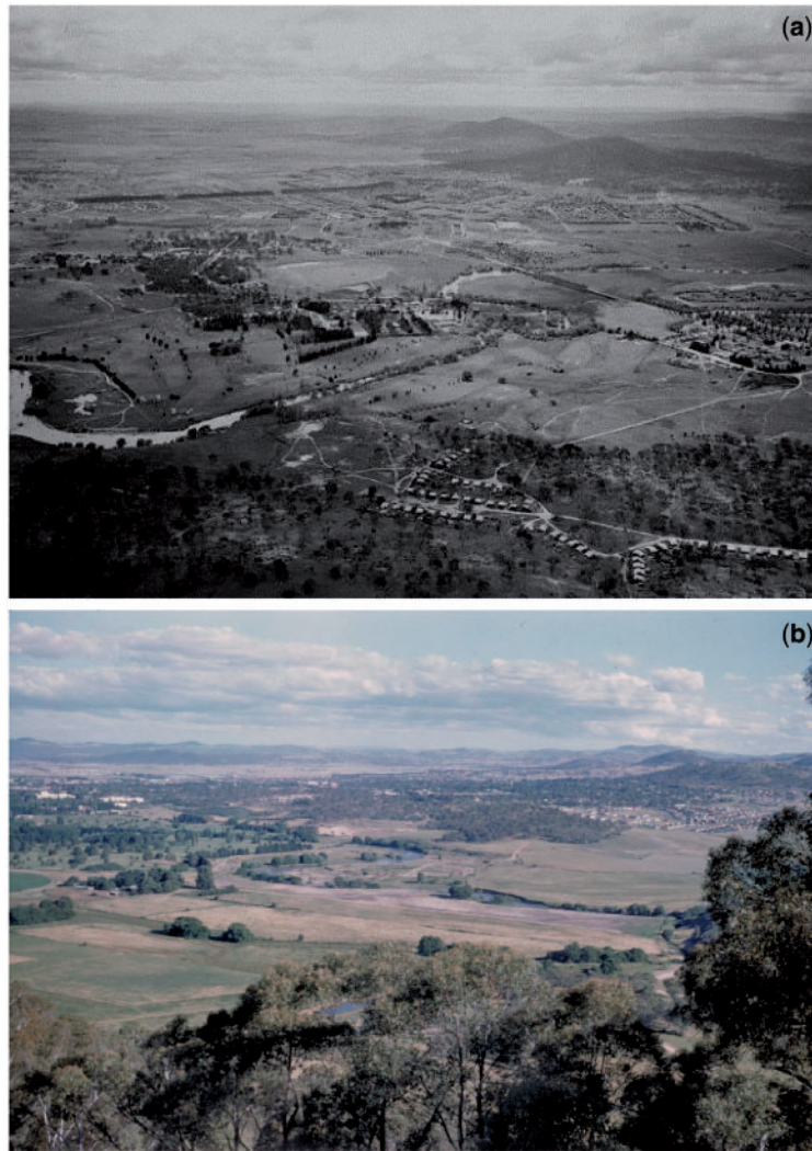
Figure 7: Changing vegetation in the mid to late 20th century. (a) Acton, Golf Links, 1951 with Molonglo River flowing through (future site of Lake Burley Griffin Westlake) Courtesy ACT Heritage Library, 17/10/1951, from Department of Capital Territory albums 'Pictorial Record of Canberra 1951–1953', Reference no 001420. (b) View of Molonglo River flowing through West Lake area prior to the construction of Lake Burley Griffin (pre-1964) from Black Mountain, Canberra. Courtesy National Library of Australia PIC P2214/321 Photograph by Richard Clough (1921–2014). Retrieved April 23, 2018, from http://nla.gov.au/nla.obj-143765195
