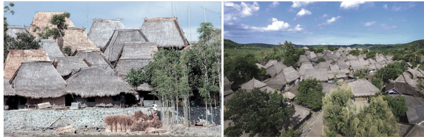
Figure 4. The roof of the traditional houses in Sade hamlet
