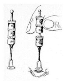
Figure 1-1 Applanation tonometry by Alexei Maklakoff, circa 1885 [10]
