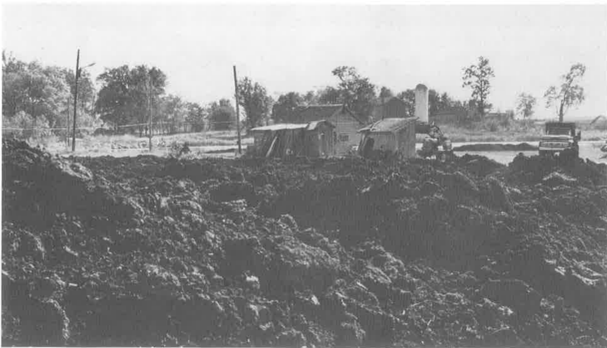
Figure 8. Excavated peat moss deposit and stockpile of Filbrun Peat Moss.
