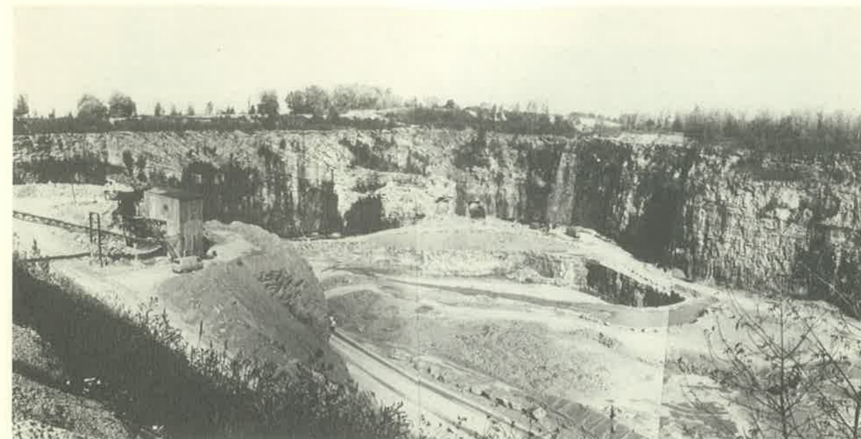
Figure 5. Lapel quarry of Martin Marietta Aggregates, Central Division.
