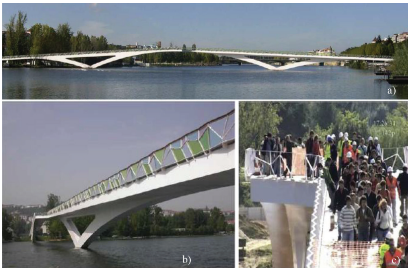
Figure 2: (a) General view of Pedro e Inês footbridge; (b) Perspective of the footbridge and (c) experimental lateral lock-in pedestrian test on this footbridge [4, 5].
